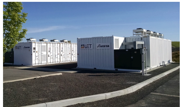
A 1 MW/4MWh vanadium flow battery operating in Pullman, WA PHOTO: Wikimedia Commons
