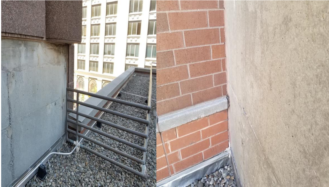
Overhang Encroachment, and butt joint without separation.
