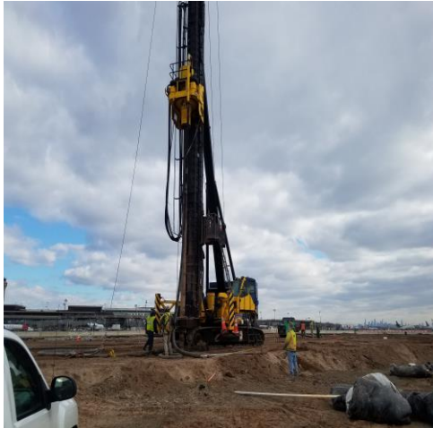
Pile drilling rig at Newark Airport. A rig of this size is necessary to drill to sufficient depth for the jail site. (authors
