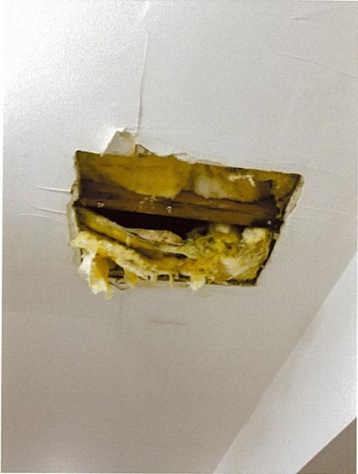
**Moldy insulation & rotting beam**
