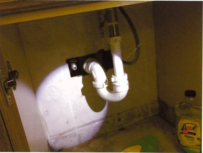
**Taken during the HPD inspection.. No violation? Missing pipe, mold, open unsealed around pipes, rat entrance, rotting**
