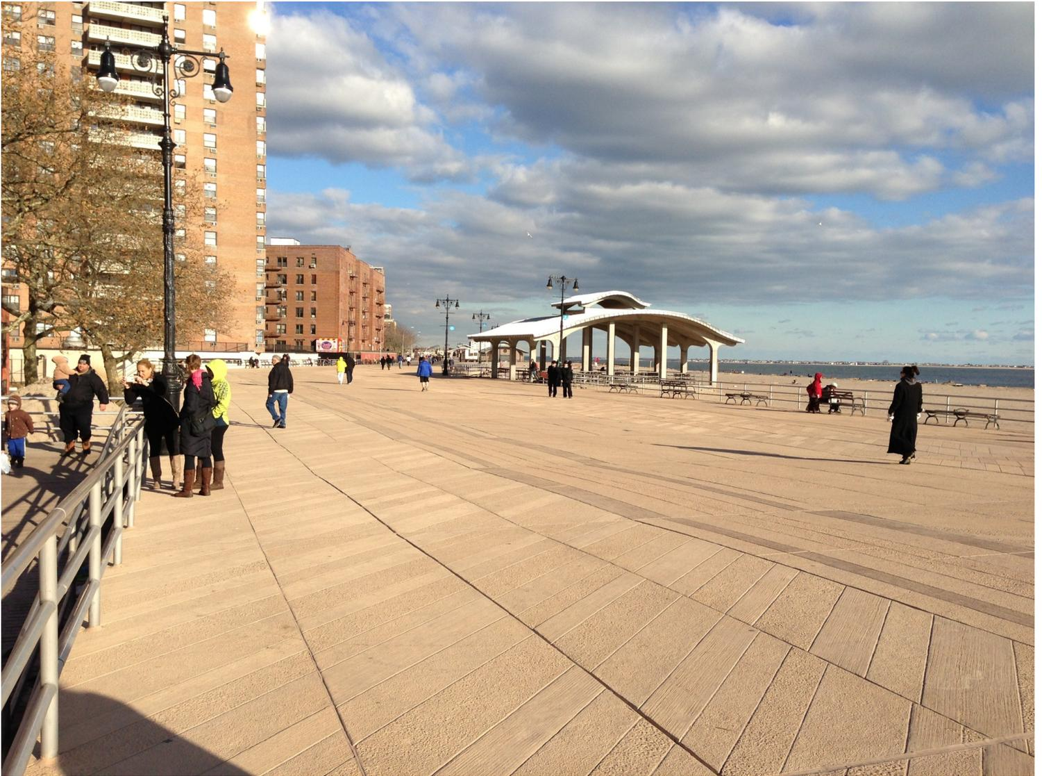
The impacts on top of the Boardwalk were even more dramatic. Here is the same concrete slab section, just west of Ocean Pkwy. The view is looking east, towards the shade pavilion. Notice that there is NO SAND on top of the concrete slab section.
