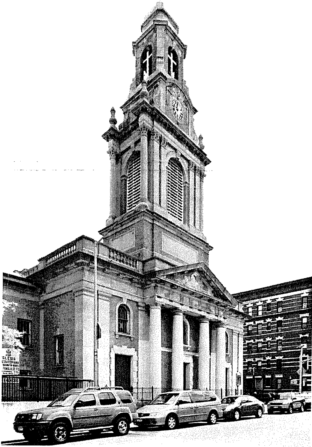
Fort Washington Presbyterian Church Wadsworth Avenue Facade Photo: Christopher D. Brazee, 2009
