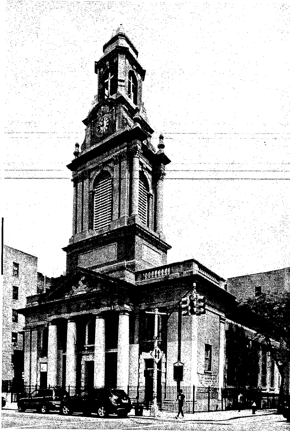
Fort Washington Presbyterian Church 21 Wadsworth Avenue (aka 21-27 Wadsworth Avenue, 617-619 West 174 th Street), Manhattan Photo: Christopher D. Brazee, 2009
