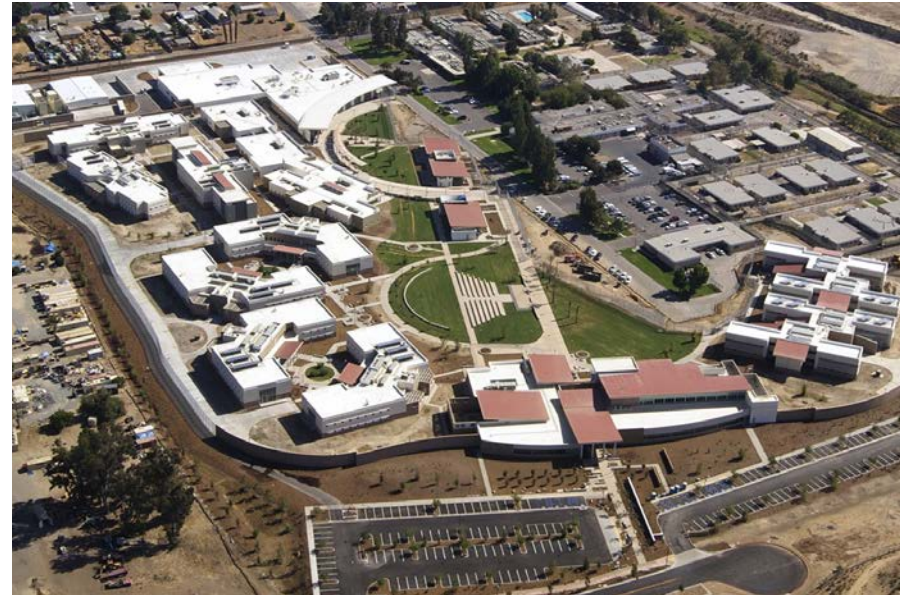
Construction of Las Colinas Women's Detention & Reentry Facility
