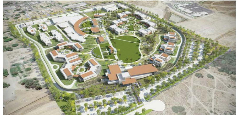
At Las Colinas Women's Detention & Reentry Facility, services are housed in separate buildings, and the inmates are escorted by deputies between the dining hall, the medical building, and the recreation and education facility.
