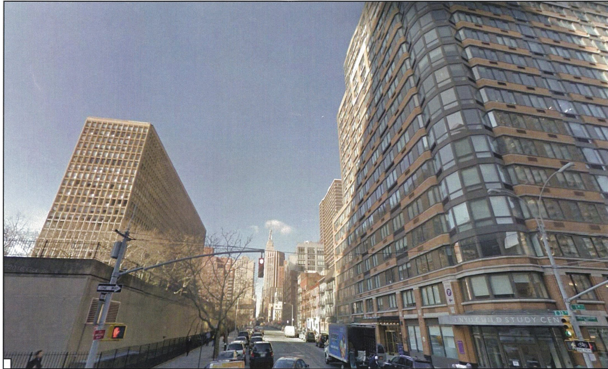
No-Action view of the project site looking west along East 33rd Street
