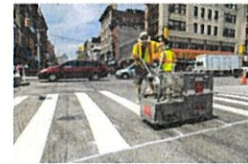
200M linear ft of markings
