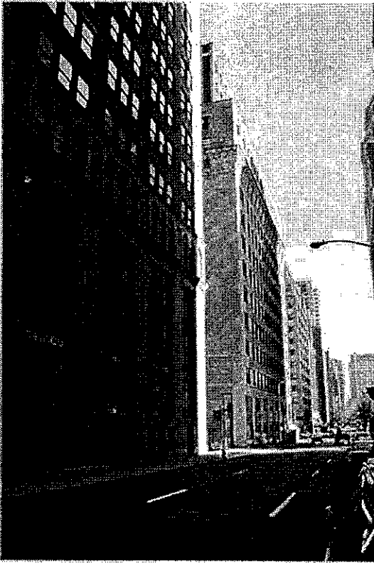
EAST 32 STREET VIEW LOOKING NORTH EAST
