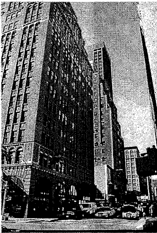
LEXINGTON AVENUE VIEW LOOKING SOUTH WEST
