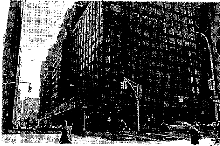
PARK AVE SOUTH VIEW LOOKING SOUTH EAST
