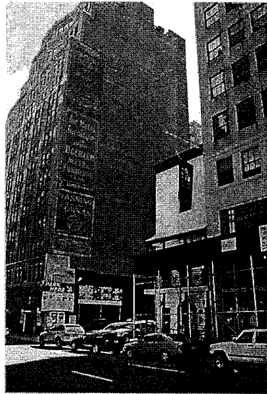
VIEW OF SITE LOOKING SOUTH EAST
