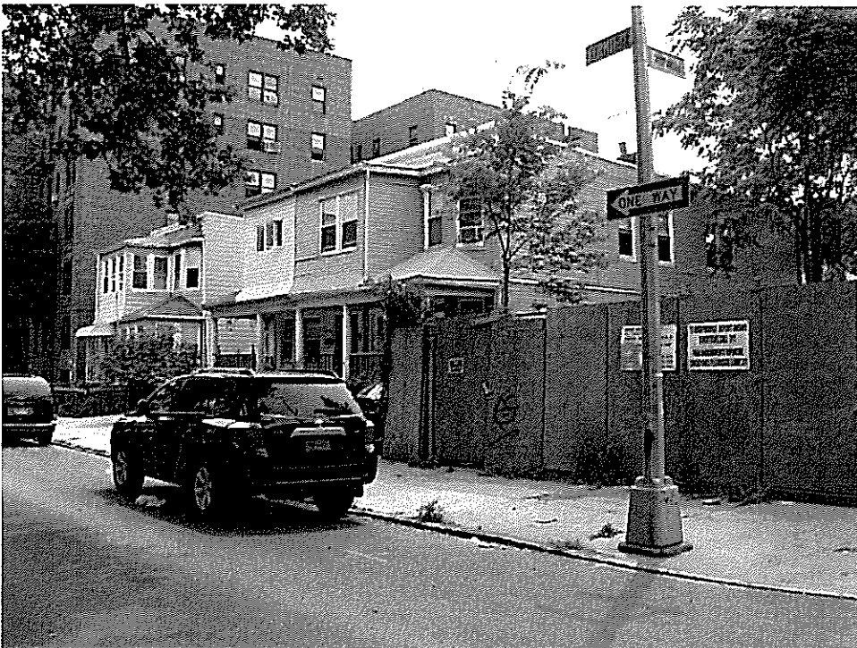
Photograph 4: Row houses and apartment building on south side of Kermit Place adjacent to project site. View looking west from intersection of Kermit Place and East 7 th Street.
