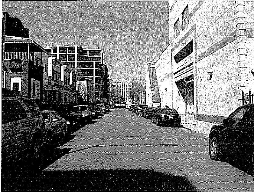
Photo 8-4: View of East 8 th Street looking north towards Caton Place. Calvary Cathedral of Praise is to the right and the apartment building under construction on Caton Place is in upper left.
