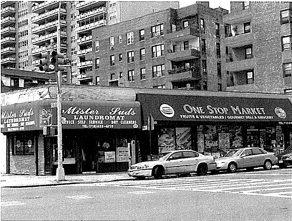
Photograph 12: Commercial buildings on south side of Caton Avenue at East 7 th Street across from project site. View looking southwest from intersection of Caton Avenue and East 7 th Street.
