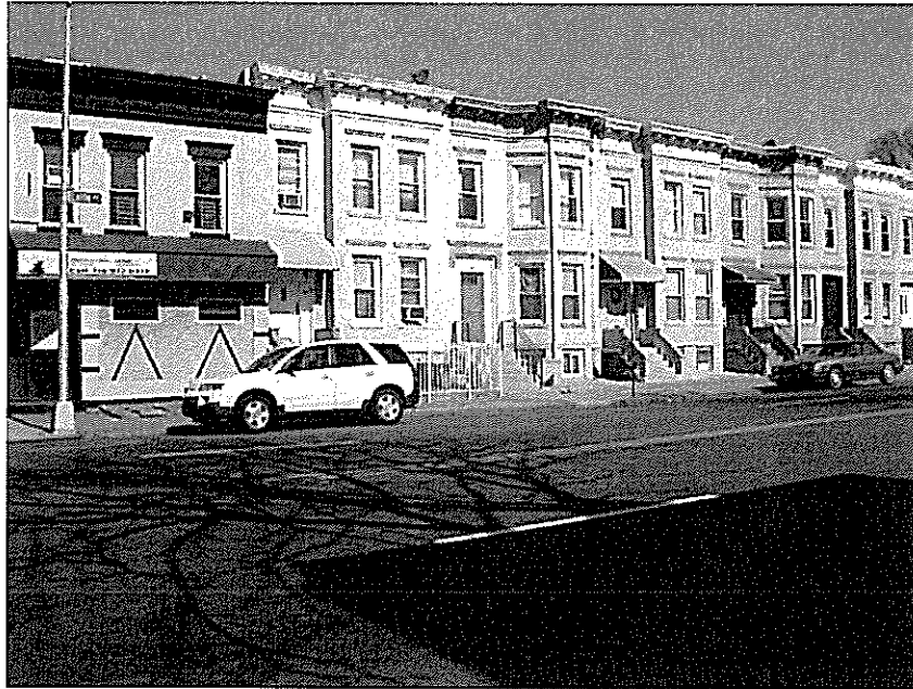
Photo 8-8: View of rowhouses on north side of Caton Avenue between Coney Island Avenue and East 8 th Street.
