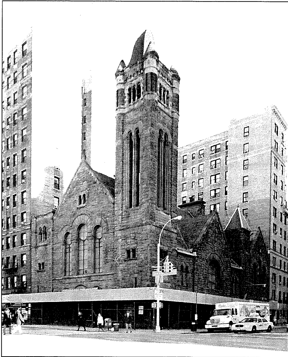
West Park Presbyterian Church, 165 West 86 th Street, Manhattan Tax Map Block 1217, Lot 1 Photo: Christopher D. Brazee, 2010
