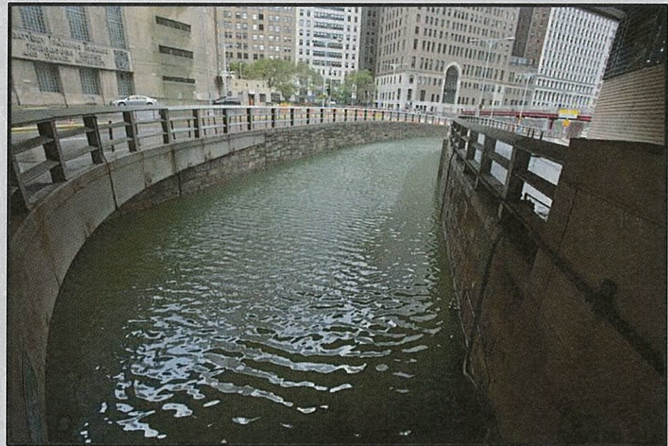
H. L. Carey Tunnel between Manhattan and Brooklyn flooded during Hurricane Sandy, October 2012
