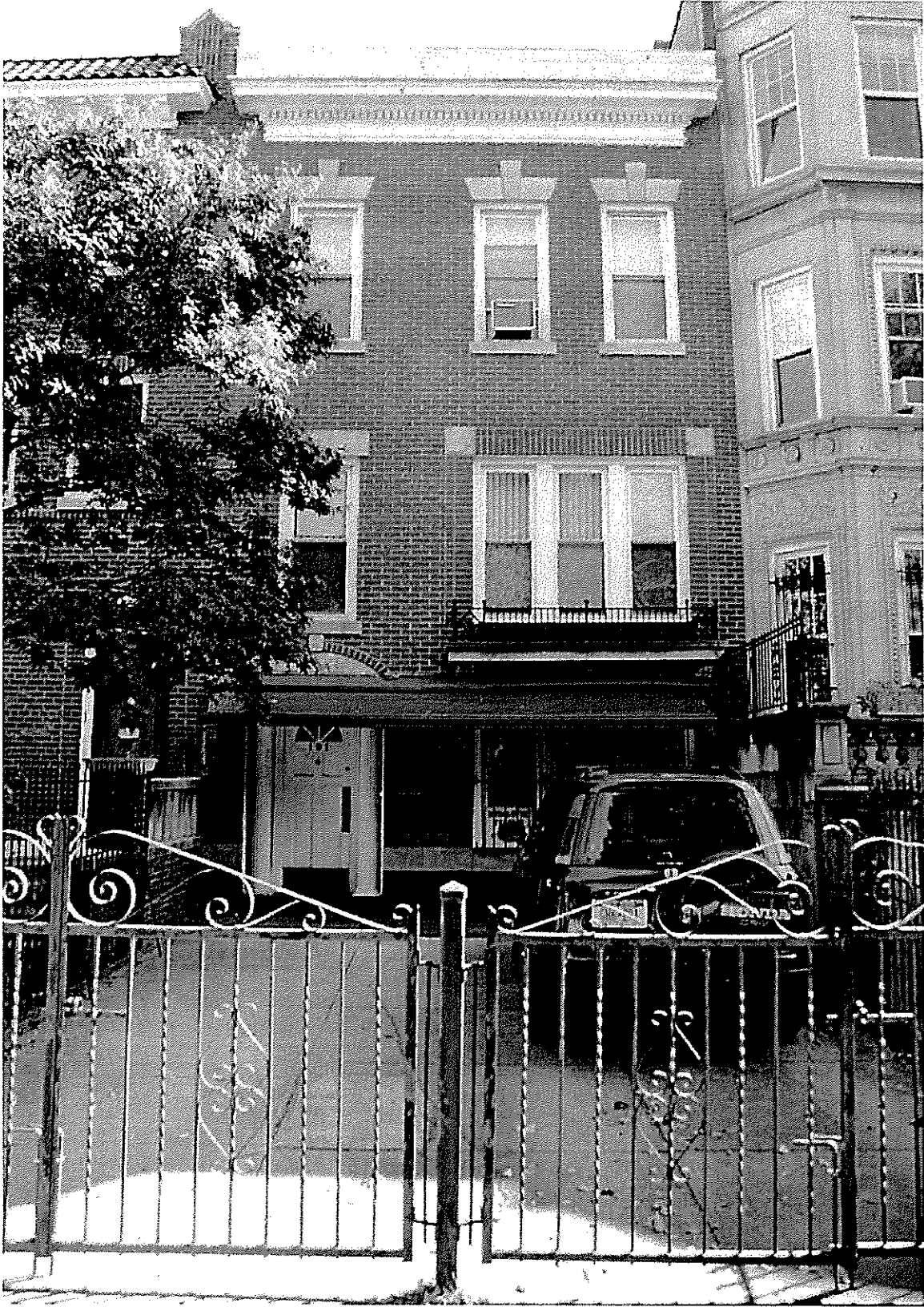
2.1.1 West (front) Facade Alterations. (Continued)
