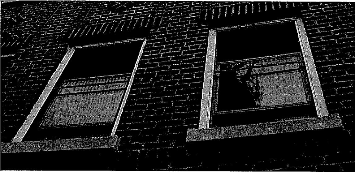
2.3.4 None of the original paint on painted elements remains and window sash and frames are pre-finished metal.
