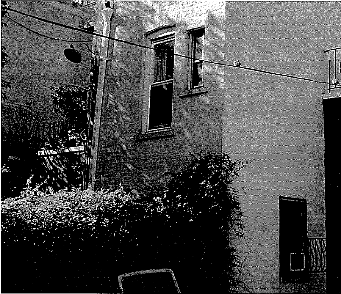
2.2.1.3 (Continued) None of the original paint on painted elements remains and window sash and frames are pre-finished metal.
