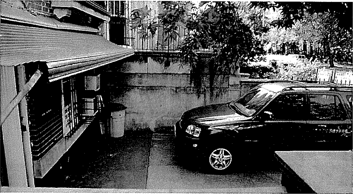
2.1.1 West (front) Facade Alterations. (Continued)
