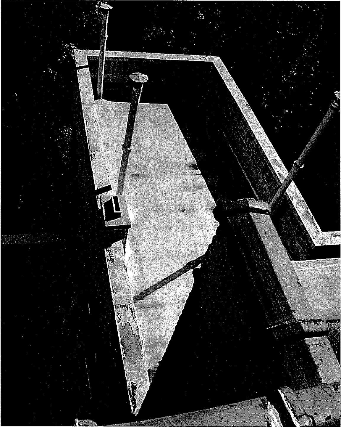
2.1.2 East (rear) Facade Alterations (Continued)
