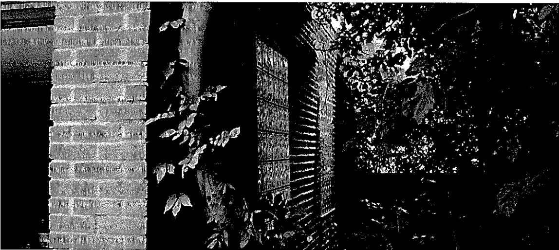
2.3.9 The garage brick lintel replaced. Glass block installed at the south wall.
