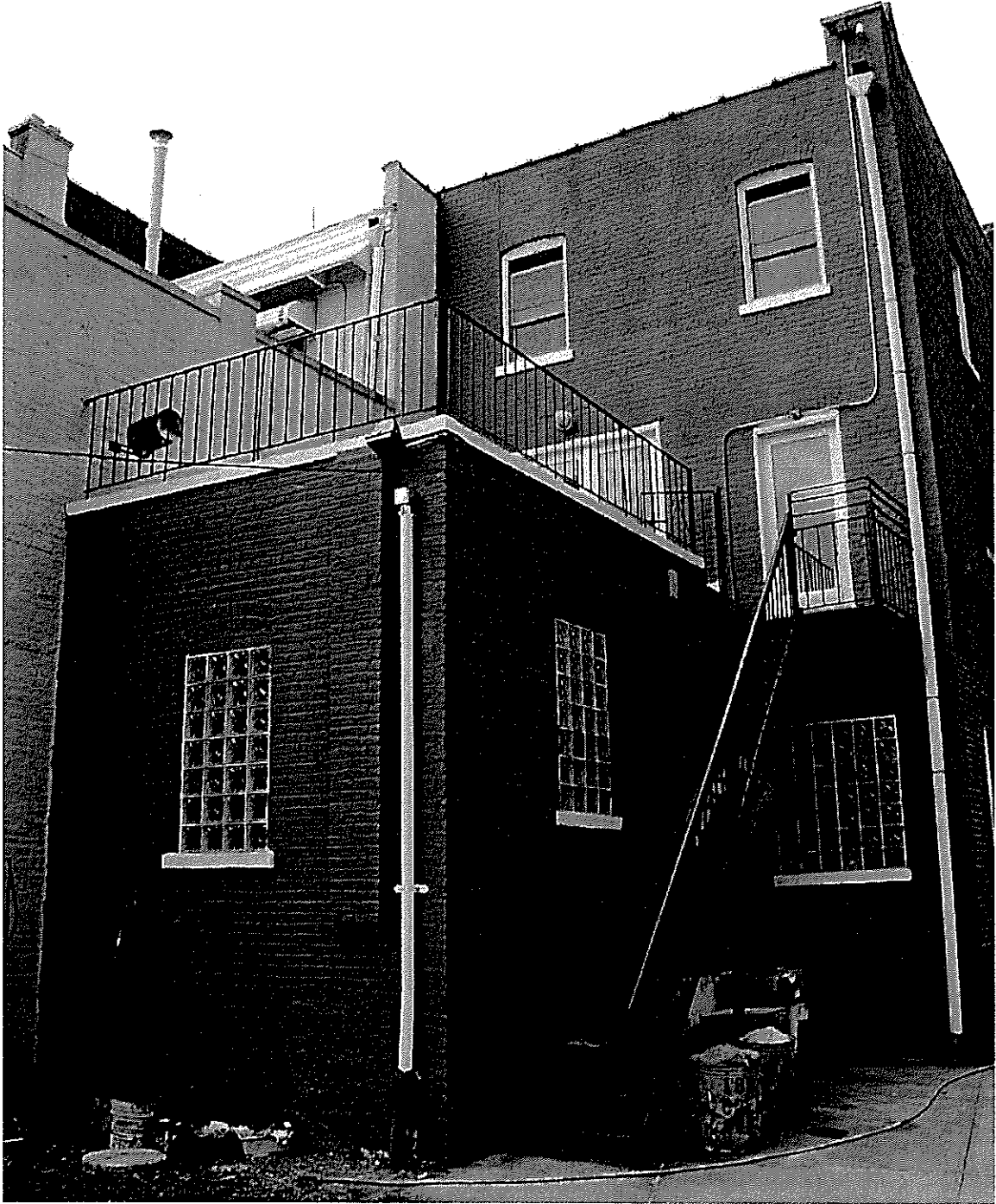
2.2.2 East Facade Alterations. Facade painted; new leader; replacement sash.
