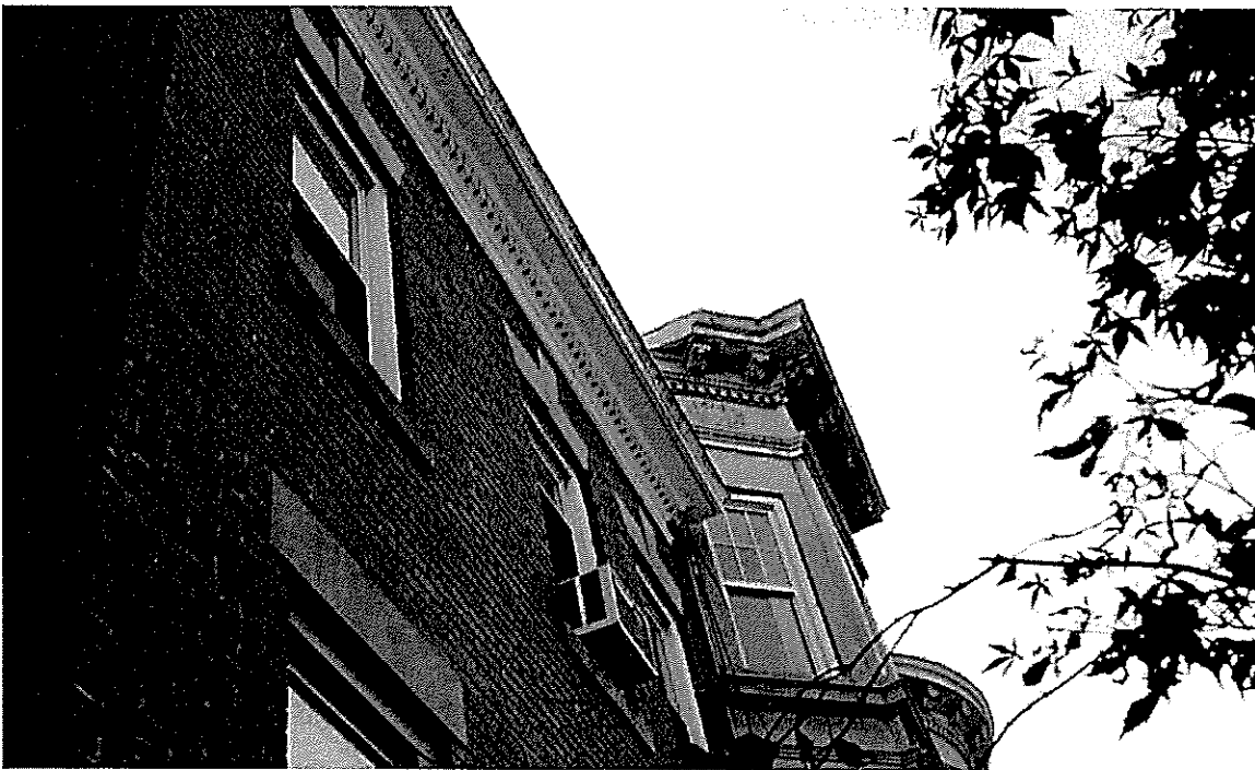
2.2.1.3 None of the original paint on painted elements remains and window sash and frames are pre-finished metal.
