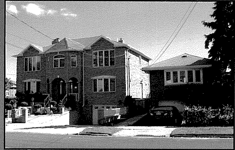
Out-of-scale detached house in an existing R2 district
