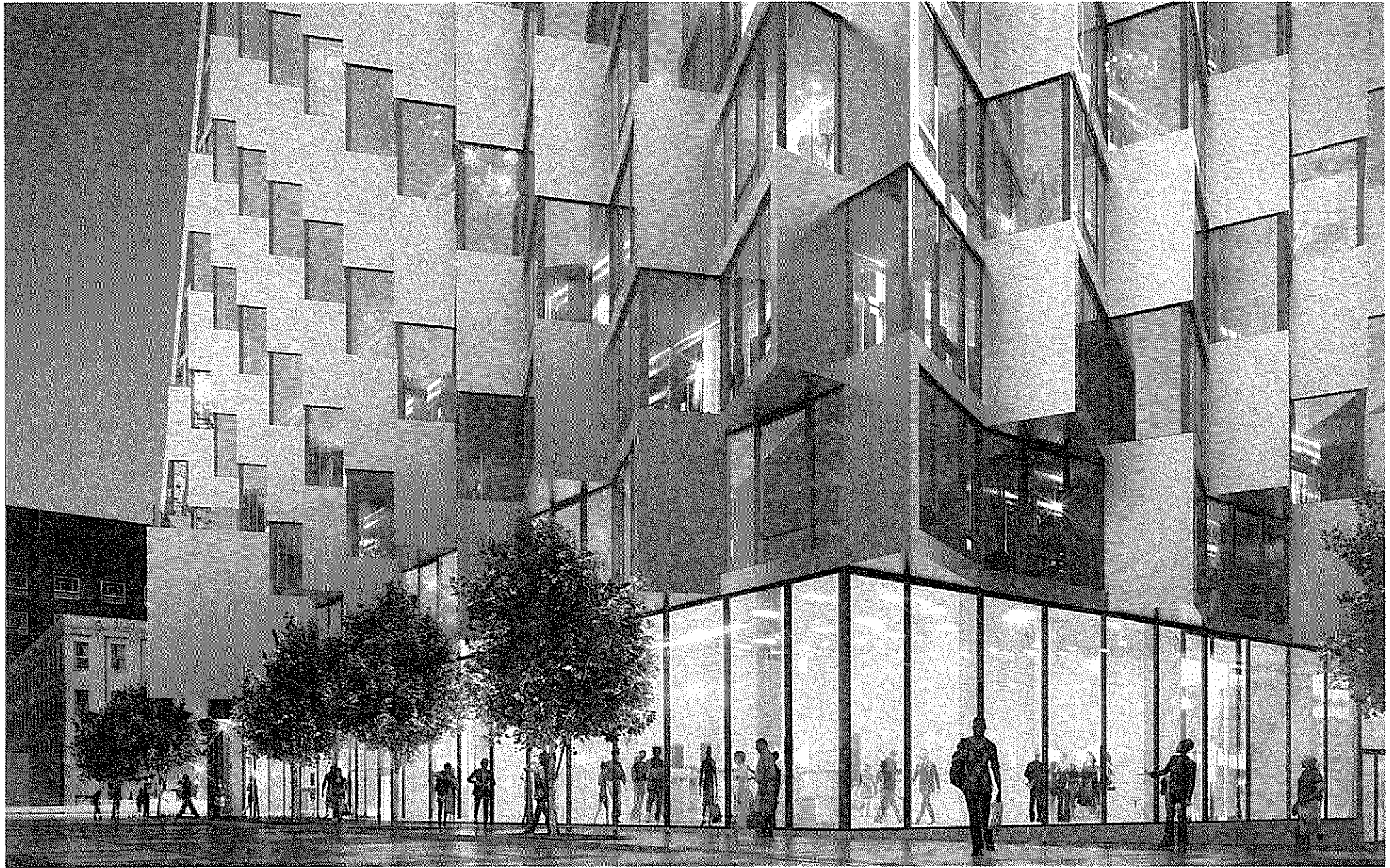
VIEW LOOKING SOUTH ON NORTH EAST CORNER
