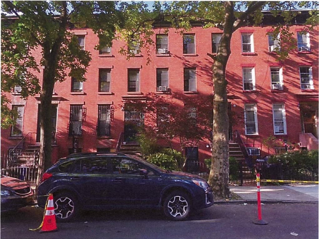
13. View of the north side of Wyckoff Street facing northeast.
