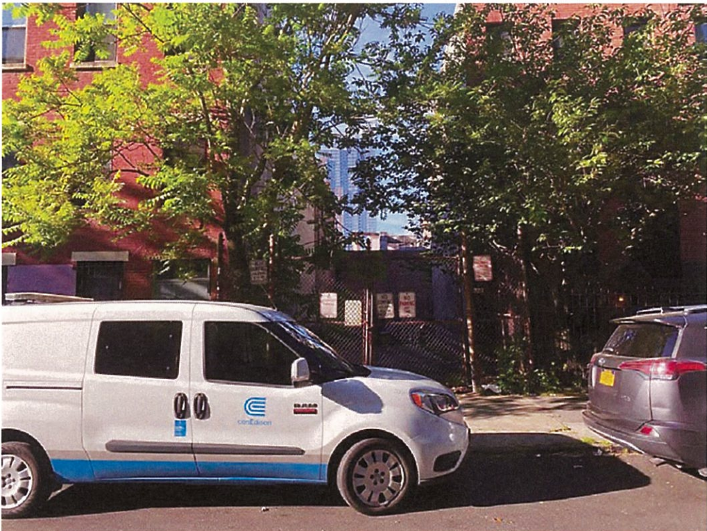
14. View of the Development Site facing northeast from Wyckoff Street.
