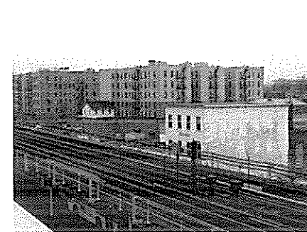
Subway Tracks along Westchester Avenue 6
