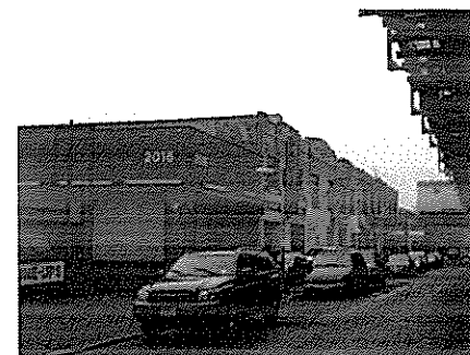
2016 Westchester Avenue looking West 9
