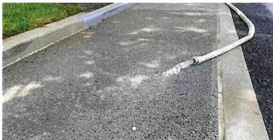
Permeable pavers and porous concrete allow water to seep in between the paving materials and be absorbed into the ground. DEP installs porous concrete in parking lanes in residential neighborhoods.
