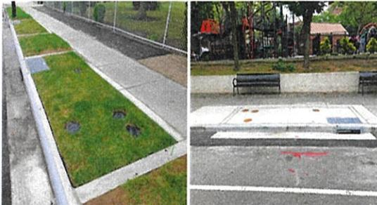
Infiltration basins are designed to store and absorb rainwater into the ground below, but at sidewalk level they have a walkable surface that blends into the surrounding conditions.
