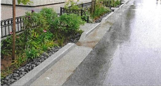
Rain gardens resemble typical curbside tree beds but are engineered to capture and store up to 2,500 gallons of rainwater that then percolate into the ground, preventing flooding.
