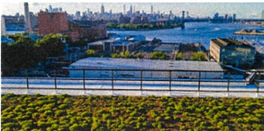
Green roofs are made up of a top vegetative layer that grows in an engineered soil, which sits on top of a drainage layer. A green roof can be “intensive,” with thicker soils that support a wide variety of plants, or “extensive,” covered in only a light layer of soil and minimal vegetation.
