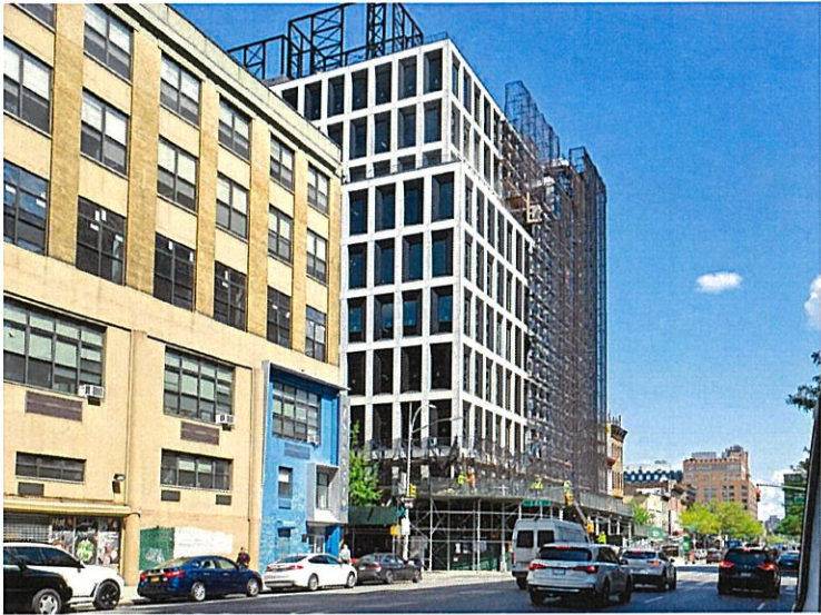
4. View of the Development Site facing north from Third Avenue between East 120th and East 121st Streets.
