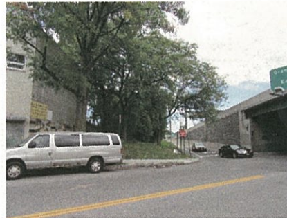
View of the Site facing northeast From 30 th Avenue
