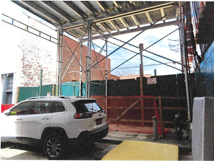
1. View of the Site facing northwest from 91st Avenue.
