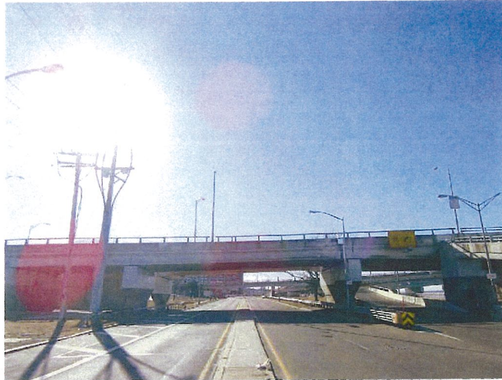
19. View of Beach Channel Drive facing southwest from Beach 92nd Street.
