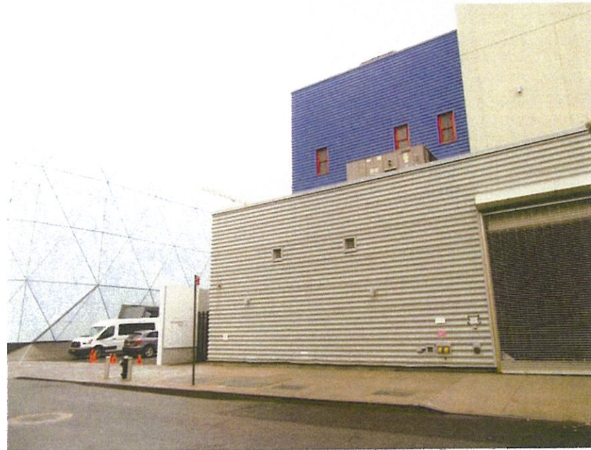
28. View of the northwest side of 37th Street facing west from the Project Area.
