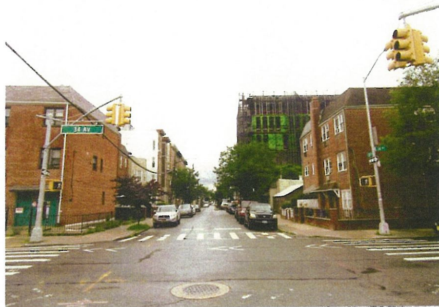
18. View of 37th Street facing southwest from 34th Avenue (Project Area at left).
