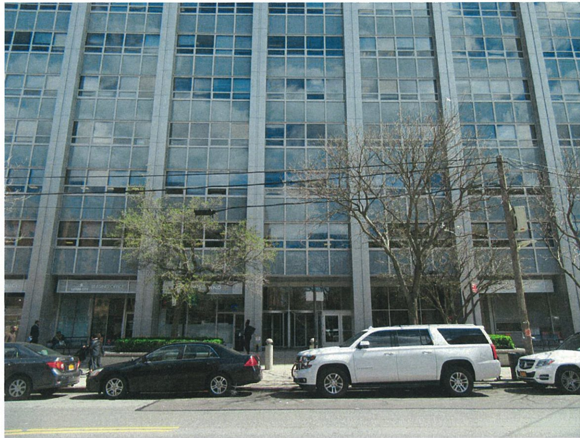
10. View of the Site facing east from Junction Boulevard.
