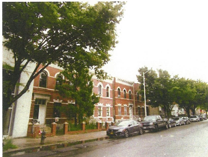
1. View of the Project Area facing north from 38th Street.
