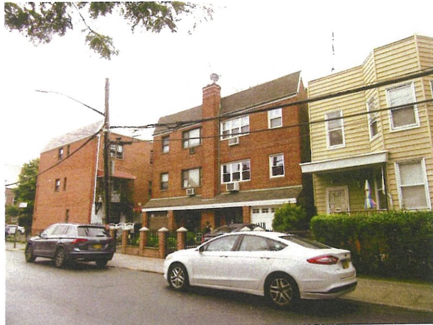
22. View of the Project Area facing east from 37th Street.
