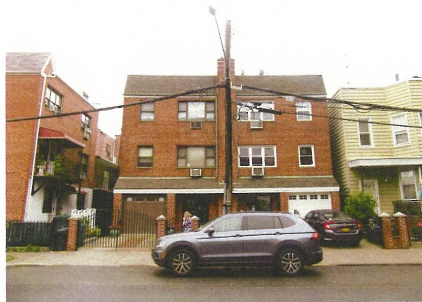
21. View of the Project Area facing southeast from 37th Avenue.
