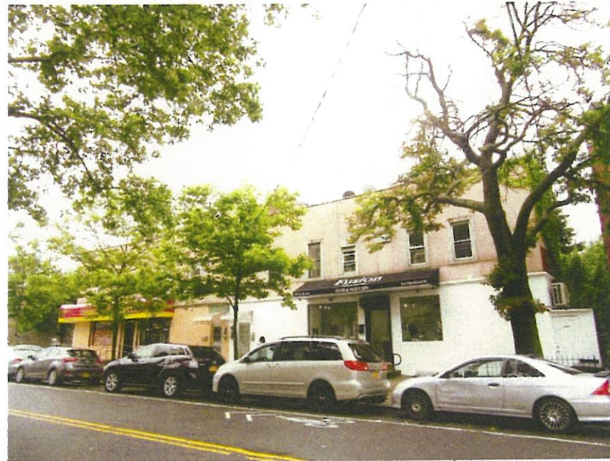
16. View of the Project Area facing south from 34th Avenue.
