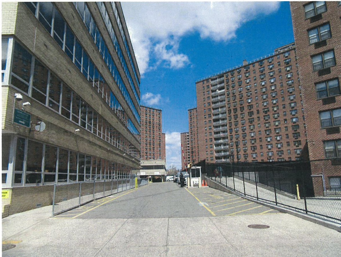
3. View of the Site facing northwest from the Horace Harding Expressway.
