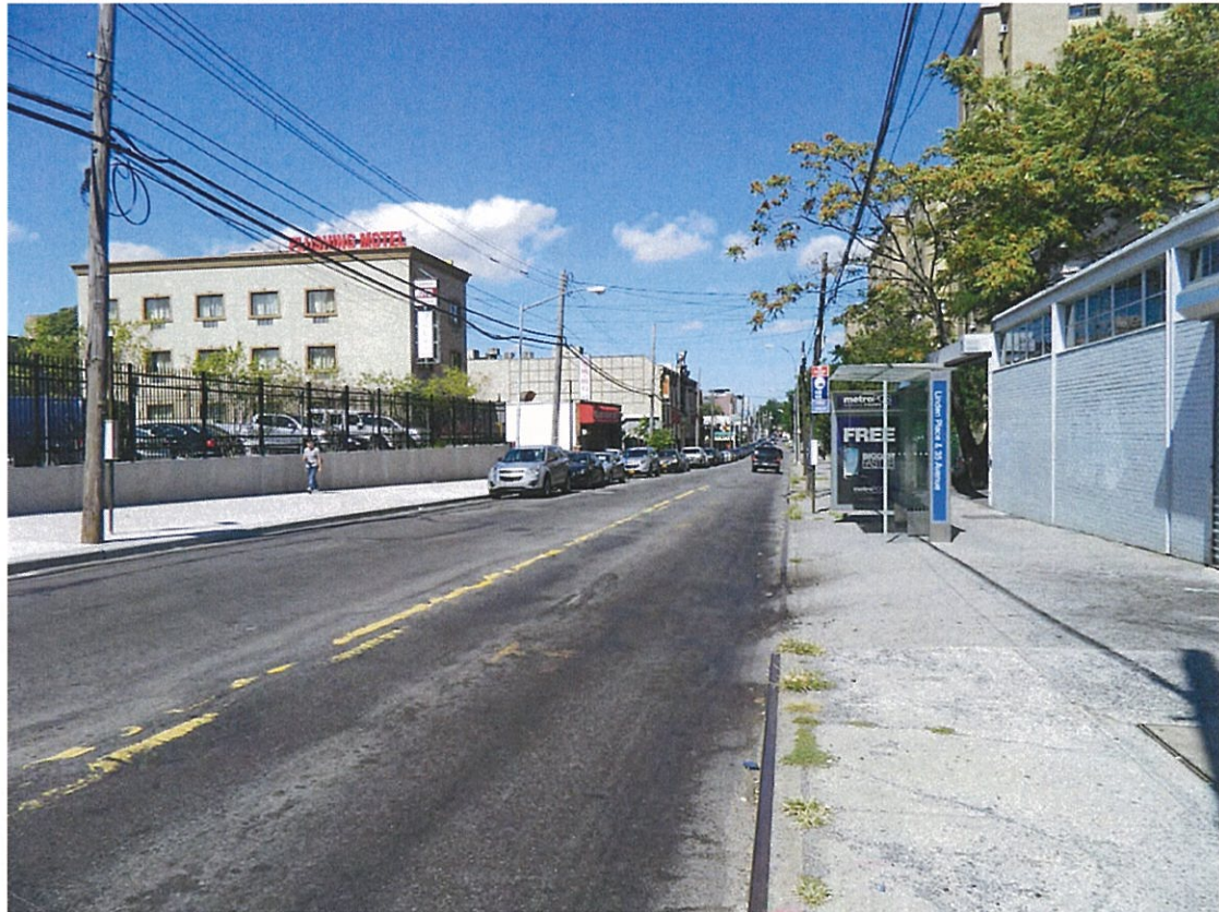
1. View of Linden Place facing north from 35th Avenue.
