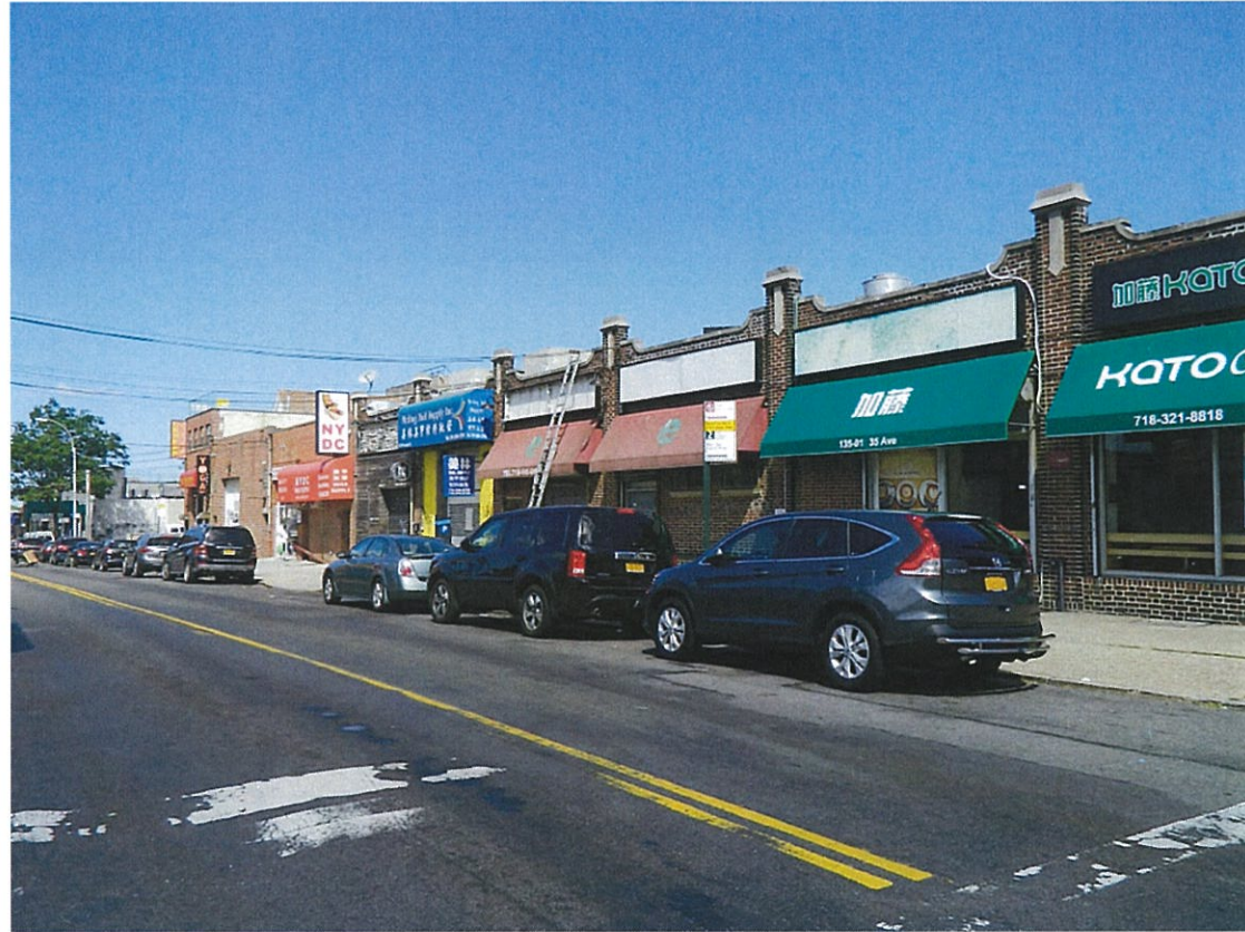
13. View of the Site facing northeast from Farrington Street.
