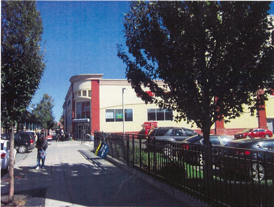
South side of Westchester Avenue looking East
