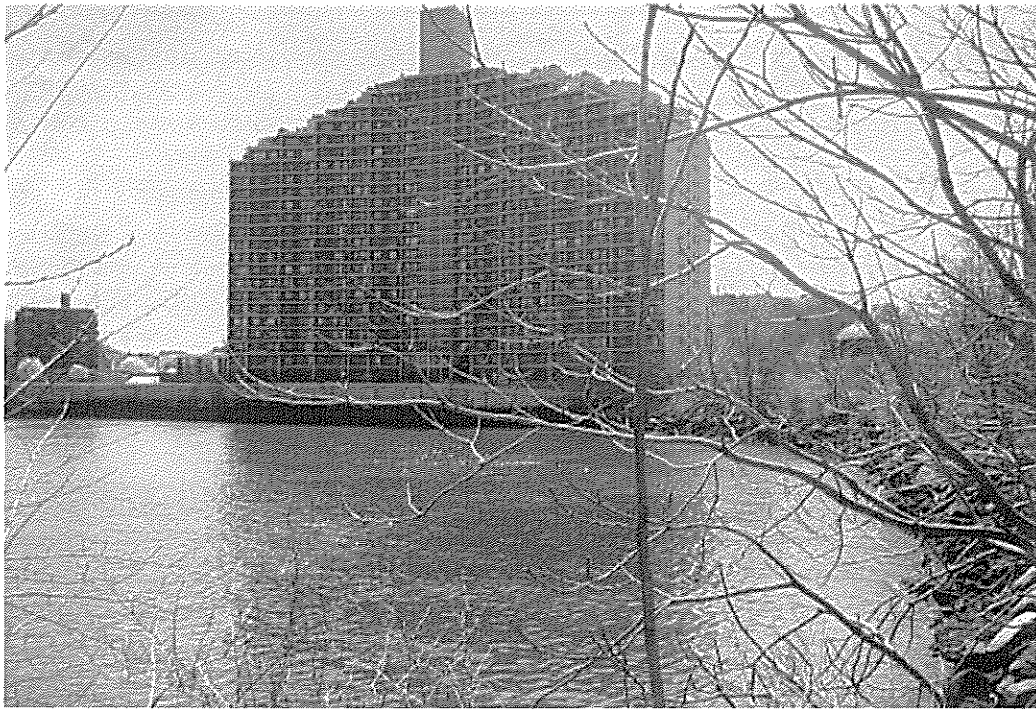
C - View Past Site to Adjacent "Shore Towers," Looking East
