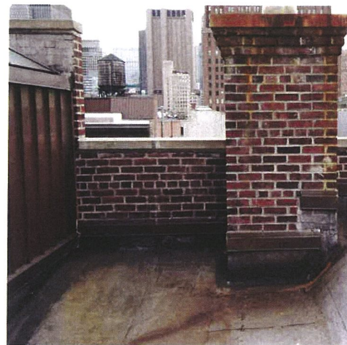
7 ROOF LEVEL PARAPET, LOOKING WEST PHOTOGRAPHED: 01.20.15
