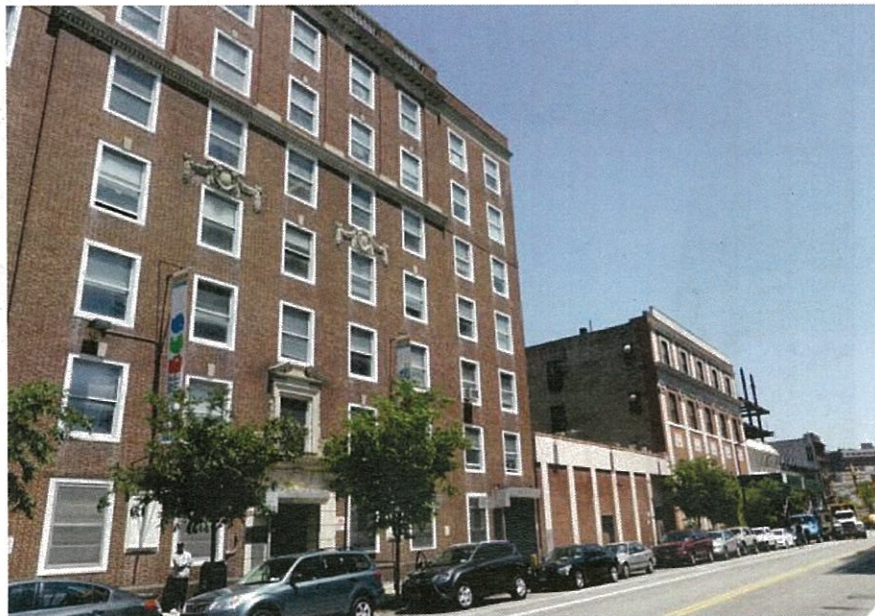
3. View East along Schermerhorn Street. Foreground shows a 7-story residential building. Photograph taken on: 06/18/2014
