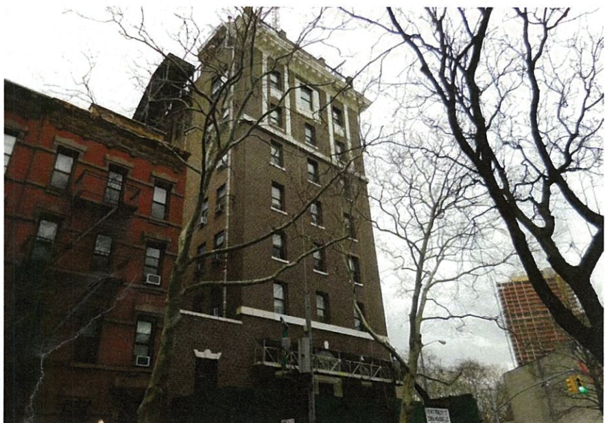
2. View East of South side of building from State Street. Photograph taken on: 02/10/2016
