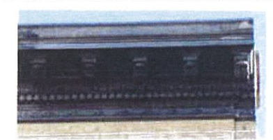
7 CORNICE DETAIL PHOTOGRAPHED: 01.06.15
