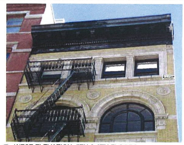
5 WEST ELEVATION, 5TH & 6TH FLOORS PHOTOGRAPHED: 01.06.15
