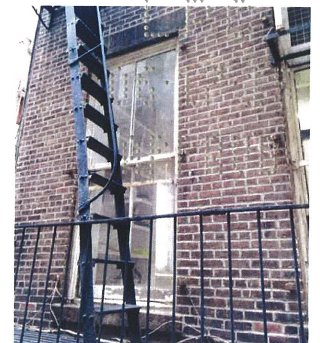
8 TYPICAL WINDOW AT EAST ELEVATION PHOTOGRAPHED: 01.20.15
