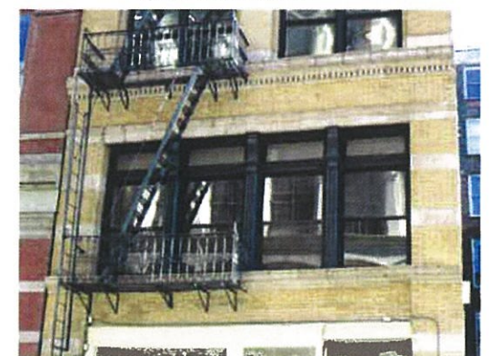
4 WEST ELEVATION, 2ND FLOOR PHOTOGRAPHED: 01.06.15
