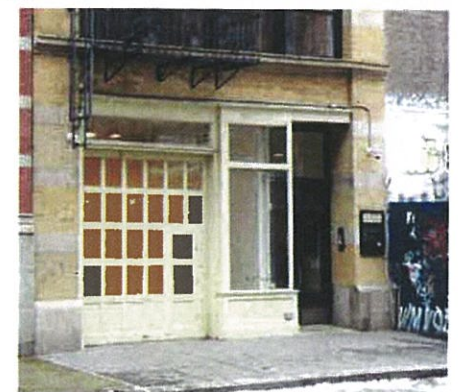
3 WEST ELEVATION, STOREFRONT PHOTOGRAPHED: 01.06.15
