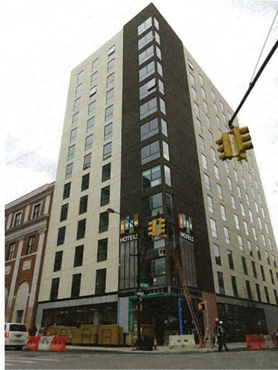
2. View North of Even Hotels at intersection between Nevins Street and Schermerhorn Street. Photograph taken on: 02/10/2016
