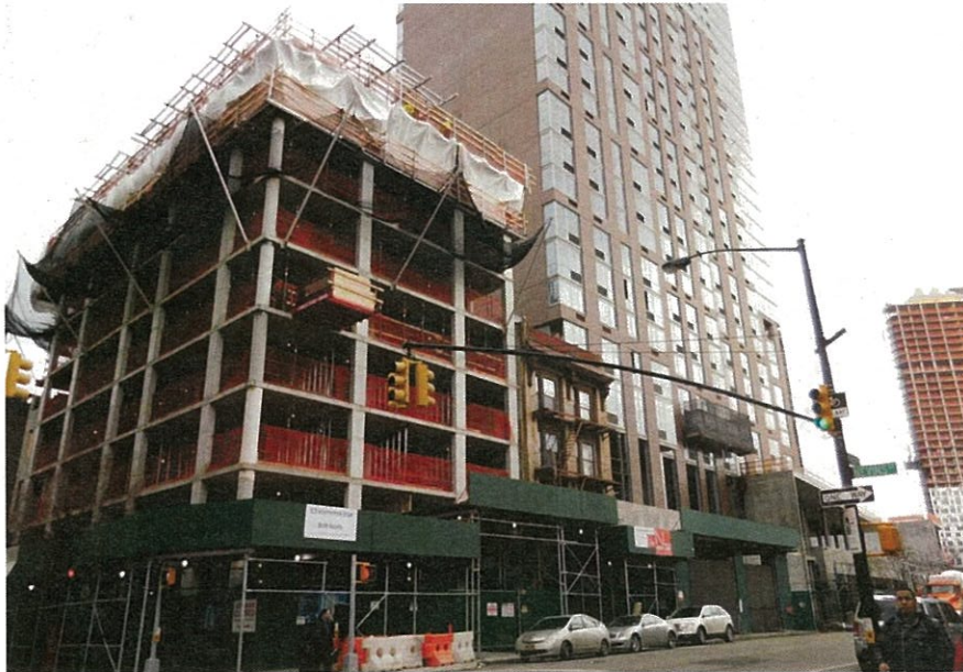
1. View East at Schermerhorn St. and Nevins St. intersection. Foreground shows two residential high-rises under construction. Photograph taken on: 02/10/2016
