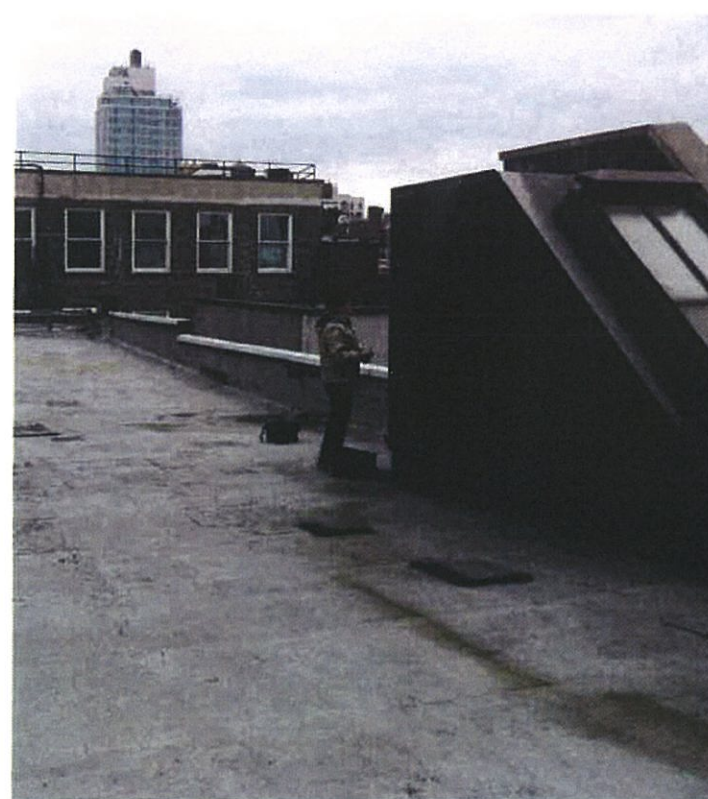
3 ROOF LEVEL, LOOKING EAST PHOTOGRAPHED: 01.20.15
