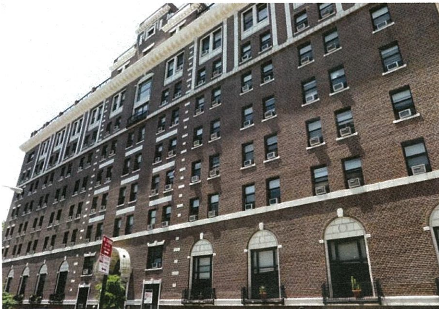
1. View West of East side of building from Nevins Street. Photograph taken on: 04/18/2014
