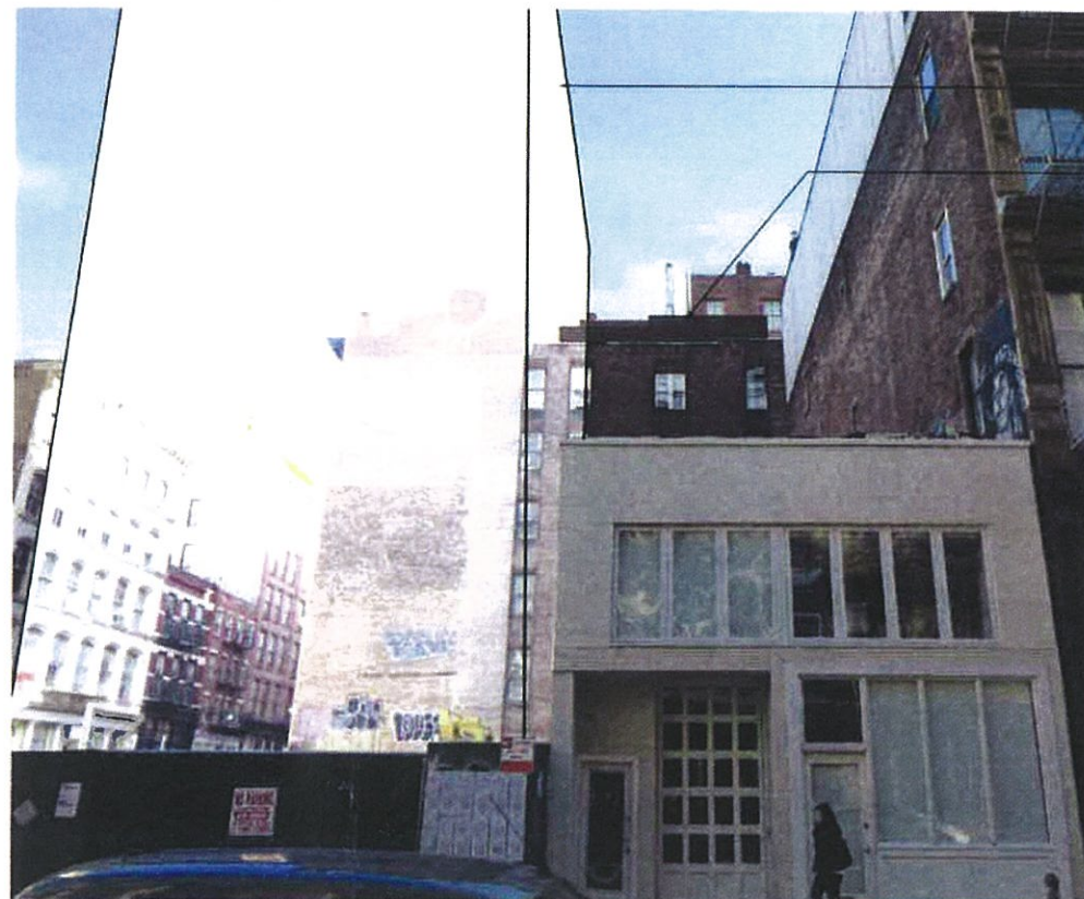
5 VIEW 06: WITH 74 GRAND BDG. OUTLINE & PROPOSED BULKHEAD MASS PHOTOSHOPPED IN SCALE: N.T.S.
