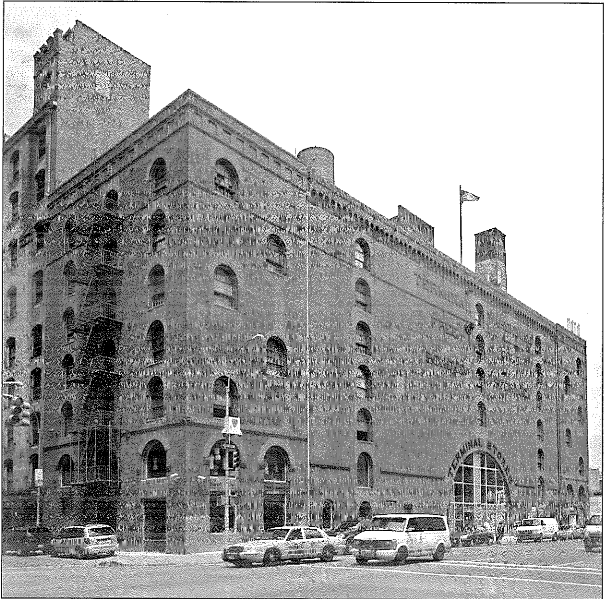
Terminal Stores Building 261 Eleventh Avenue
