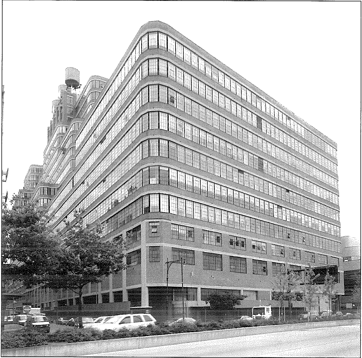
Starrett-Lehigh Building 601-625 West 26 th Street
