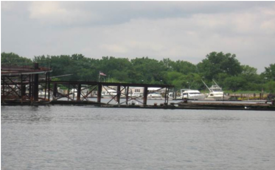
Mariners Harbor Yacht Club Bulkhead and Piers 06.27.2014
