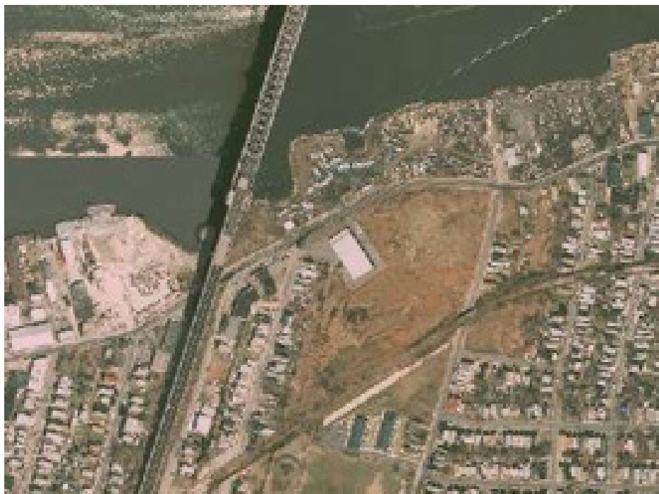
Aerial Photo of the Bayonne Bridge Port Authority Property 2007
