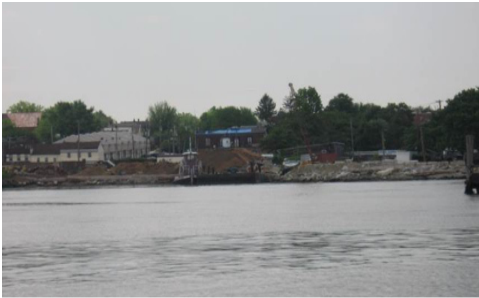
Mariners Harbor, Shoreline Erosion with some Riprap 06.27.2014
