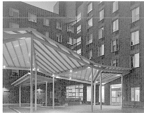
after view of canopy
