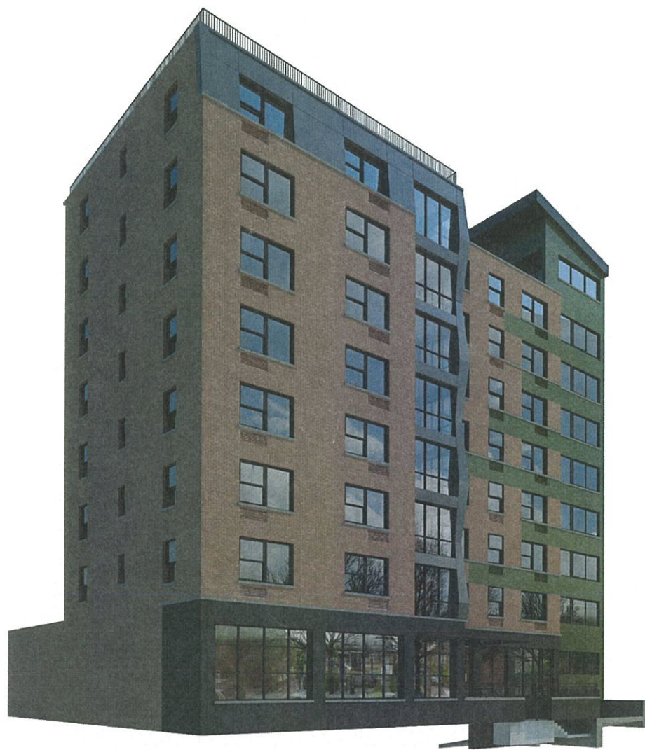
FROM WILLIAMSBRIDGE ROAD
