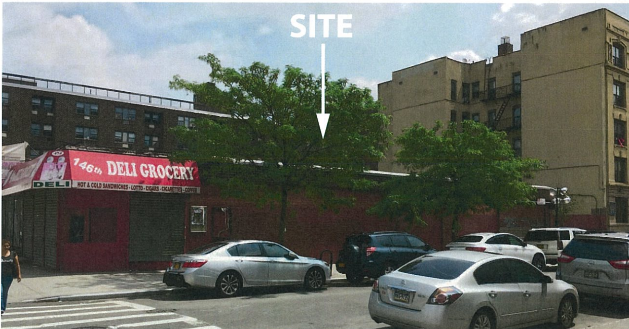
2 VIEW OF SITE LOOKING WEST ON 146th STREET JULY 17, 2018
