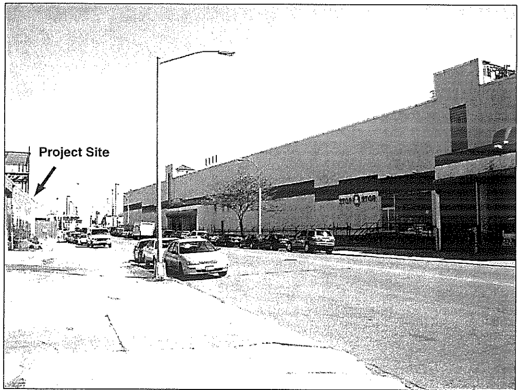
Stop and Shop storage warehouse, view northeast on 74th Street 8
