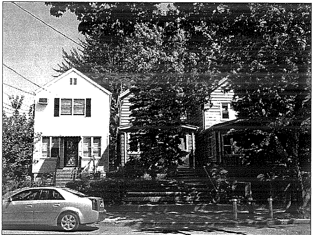
Residential buildings on project site block, view north on 57th Street 4
