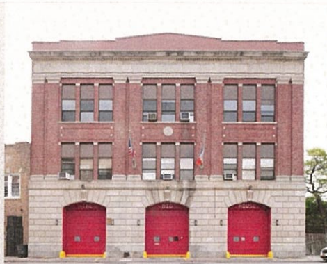
Firehouse, Engine Company 264 & 328 Hook and Ladder 134
