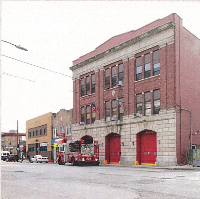
Firehouse, Engine Company 264 & 328, Hook and Ladder 134
