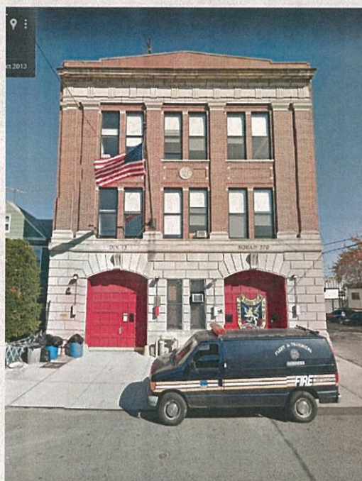
Engine Company 98 91-45 121st Street, Jamaica, Queens
