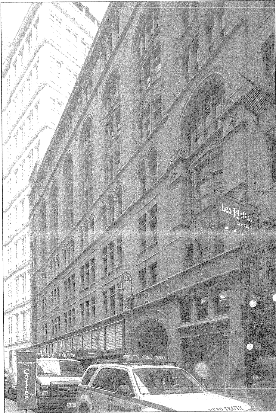
Corbin Building, John Street (South) Elevation Photo: Christopher D. Braze (2015)
