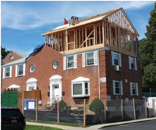
Dormer under construction on 260th Street.
