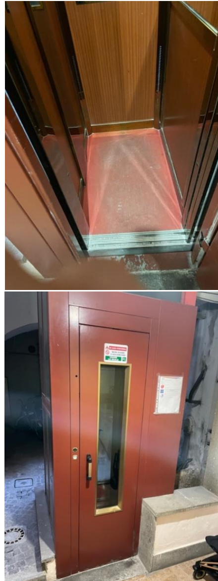
A typical installation of a small elevator in an existing building in Rome, Italy.
