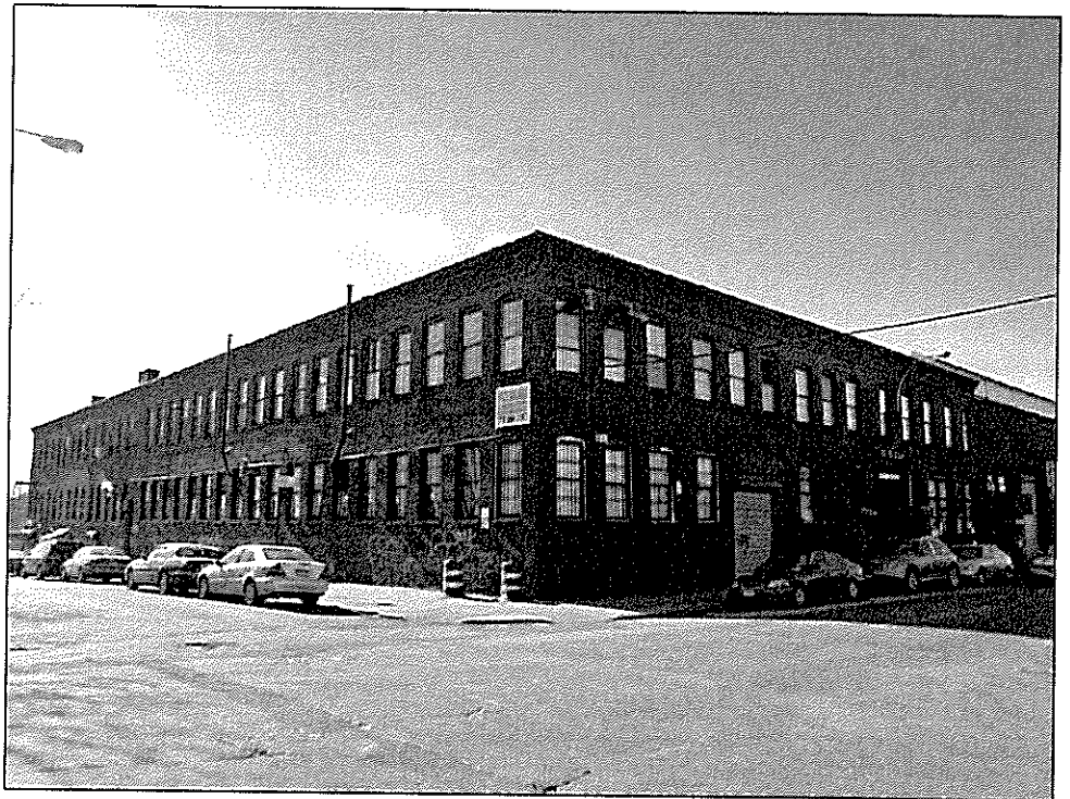
View southwest to the project site from 43rd Avenue and 97th Place 1
