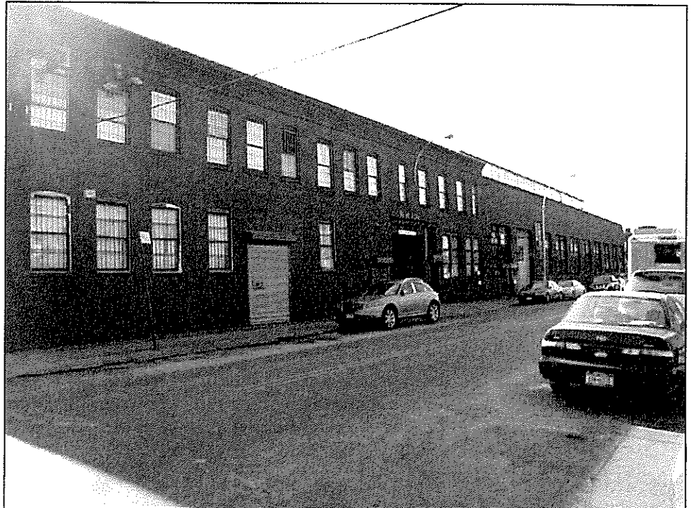
View southwest to the former Tiffany Studios Complex's 43rd Avenue facade 2
