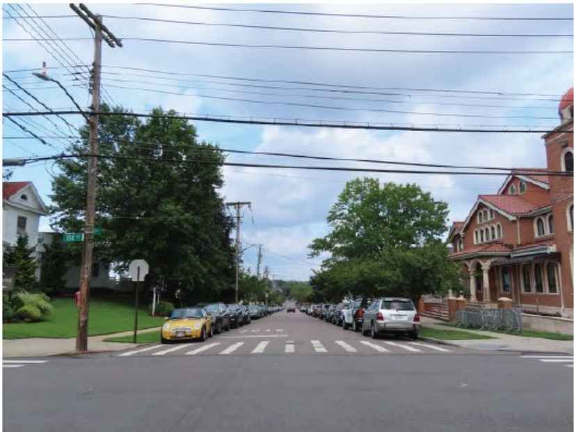
7. View of 11th Avenue facing northeast from 150th Street (Development Site at left).
