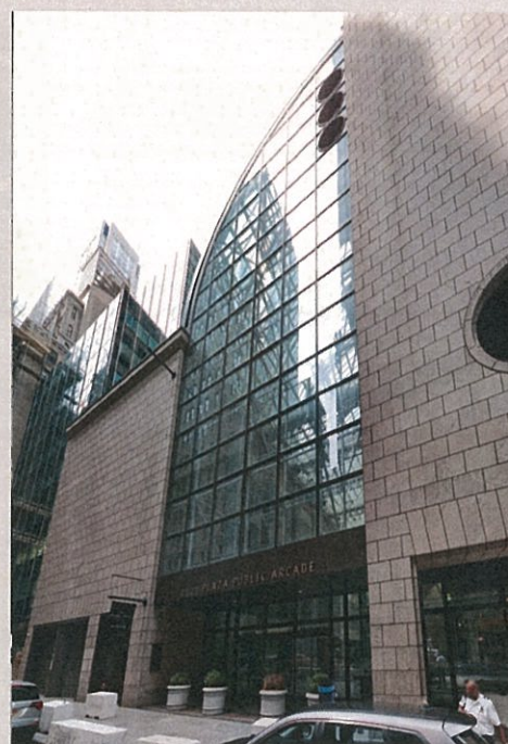
Entrance to covered pedestrian space, East 55 th Street, 2017
