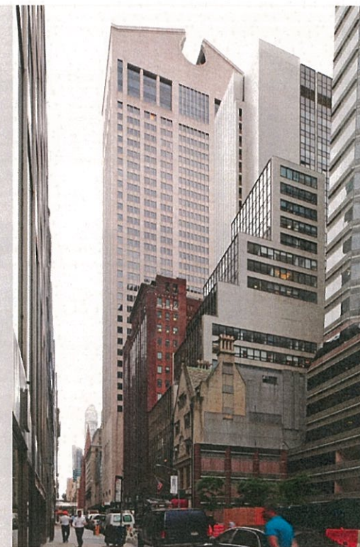
Tower viewed from west, 2018
