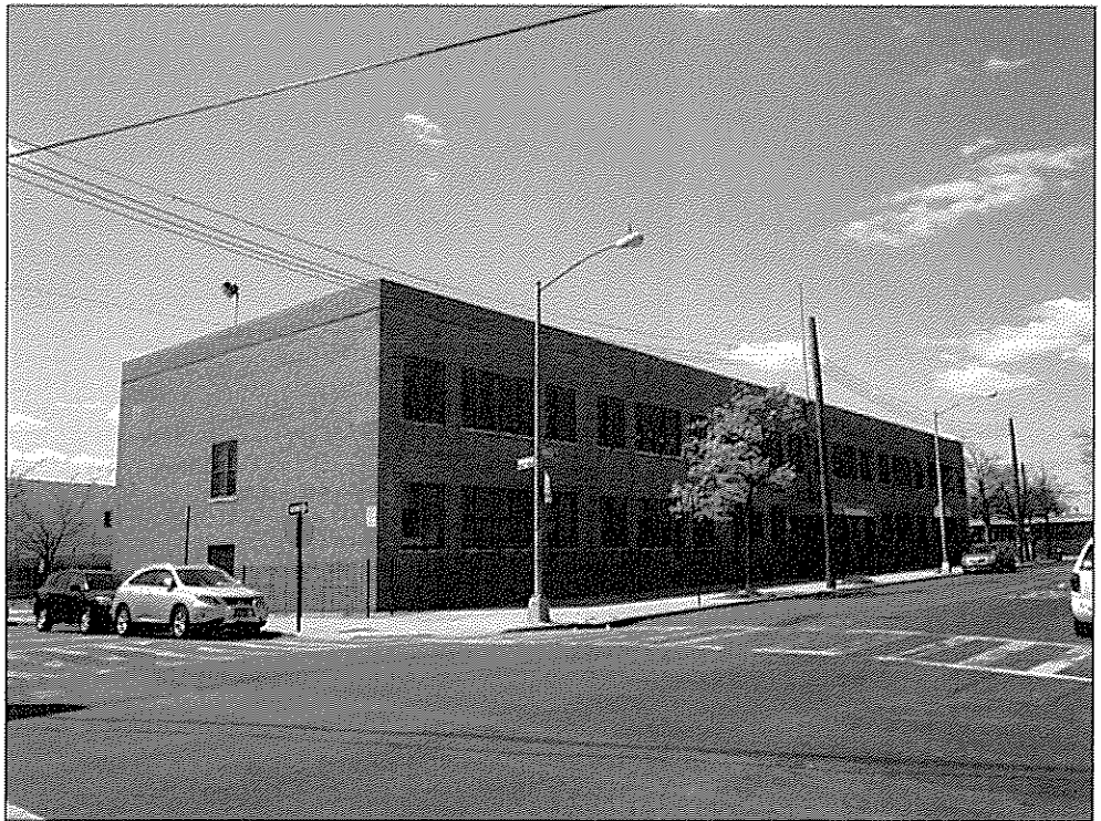
View looking west at the project site from Seneca Avenue and Stockholm Street 1
