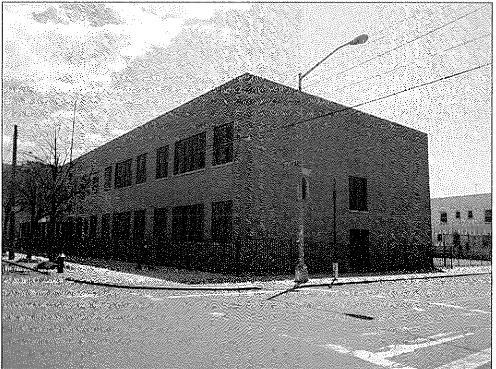
View looking southeast at the project site from Seneca Avenue and DeKalb Avenue 2
