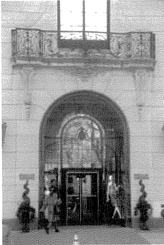
Original entrance, West 58 th Street
