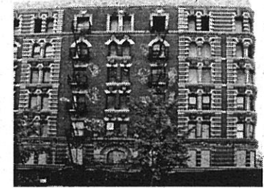
Photo 2 The current status of that building, September 2010: abandoned and unrepaired
