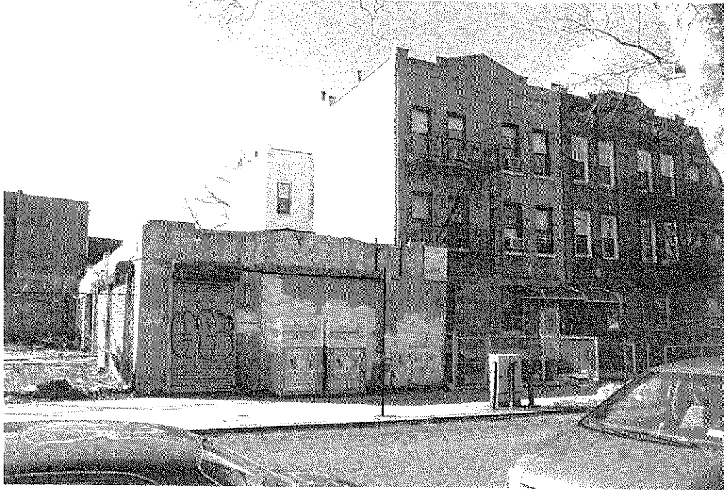
7. VIEW BUILDINGS ON 54TH STREET, NORTH OF FORT HAMILTON PARKWAY LOOKING WEST
