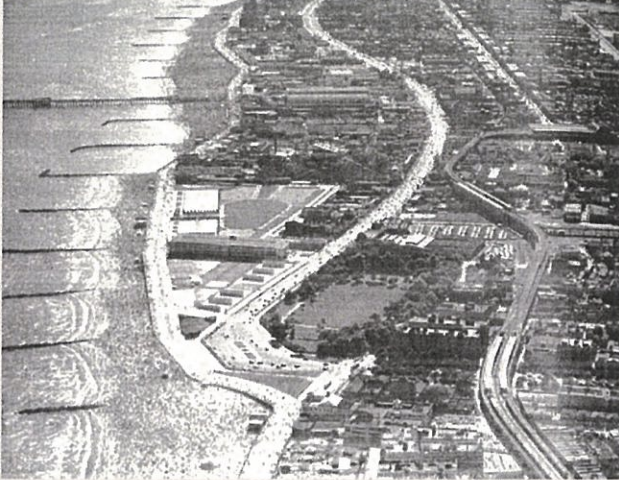
Coney Island Boardwalk prior to realignment, late 1930s Shore and Beach magazine, 1943
