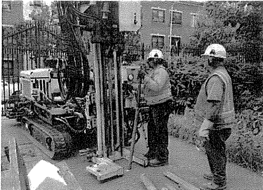
Boring machine taking soil samples from Epiphany Playground, Williamsburg
