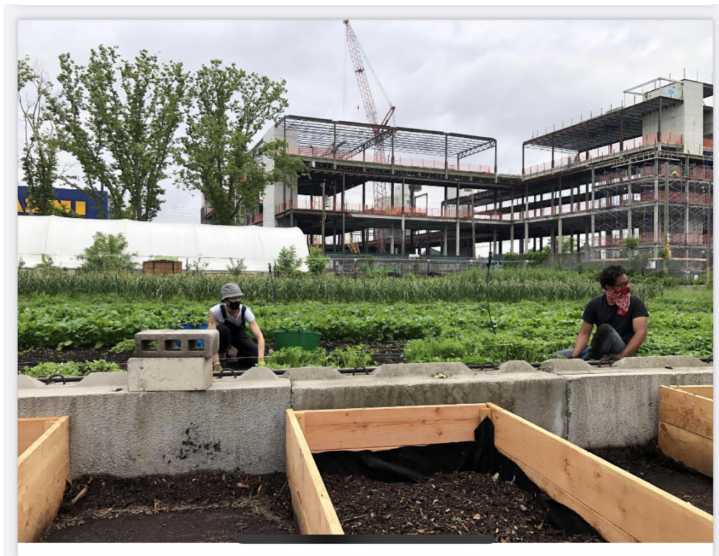
Construction of Amazon Facility next to Columbia St. Farm
