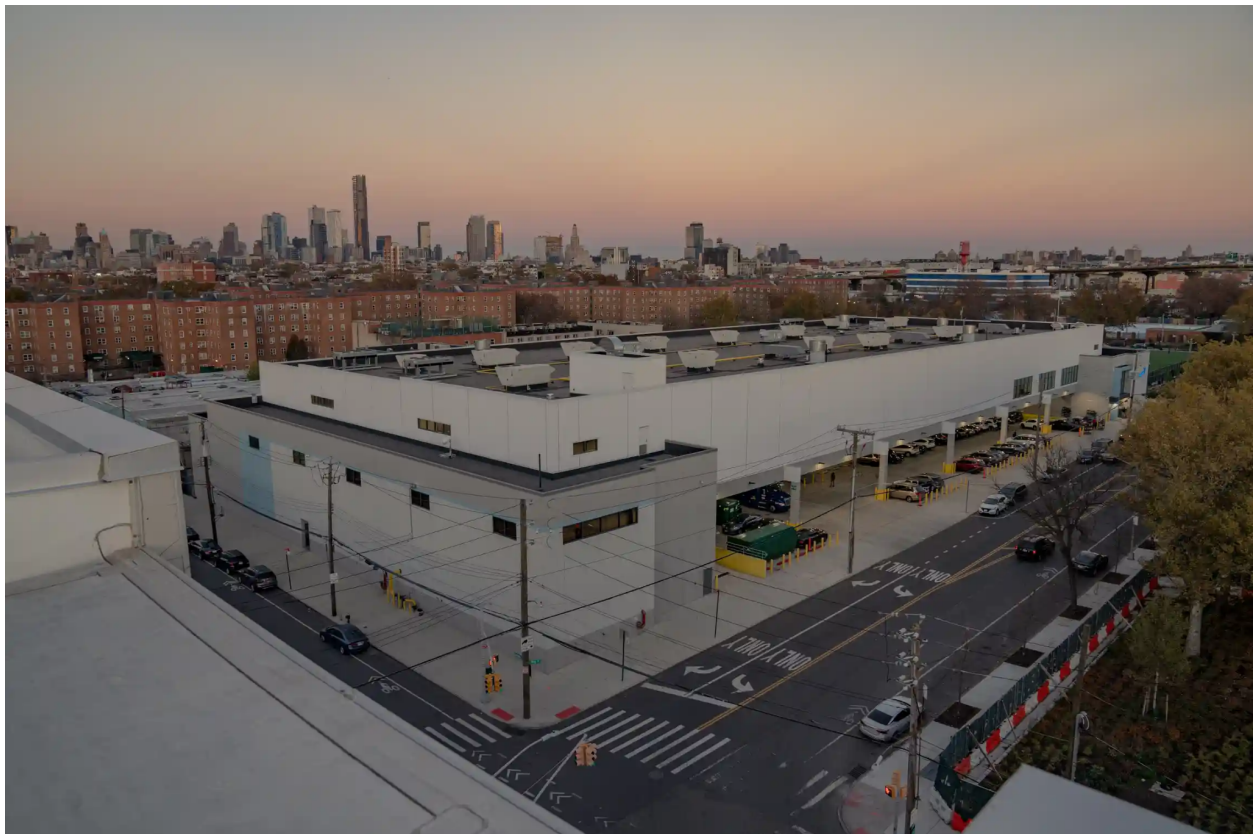
Newest Amazon facility (Red Hook Houses in background)
