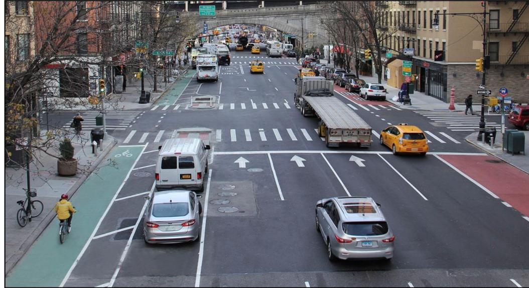
Traffic signals are coordinated to efficiently move vehicles, pedestrians, and cyclists. To best coordinate signals, adjacent intersections have the same signal cycle length, typically 60, 90, or 120 seconds. Each traffic movement is allotted a certain percentage of time in the cycle, known as a phase, based on the number of vehicles, pedestrians, and cyclists moving in each direction.
