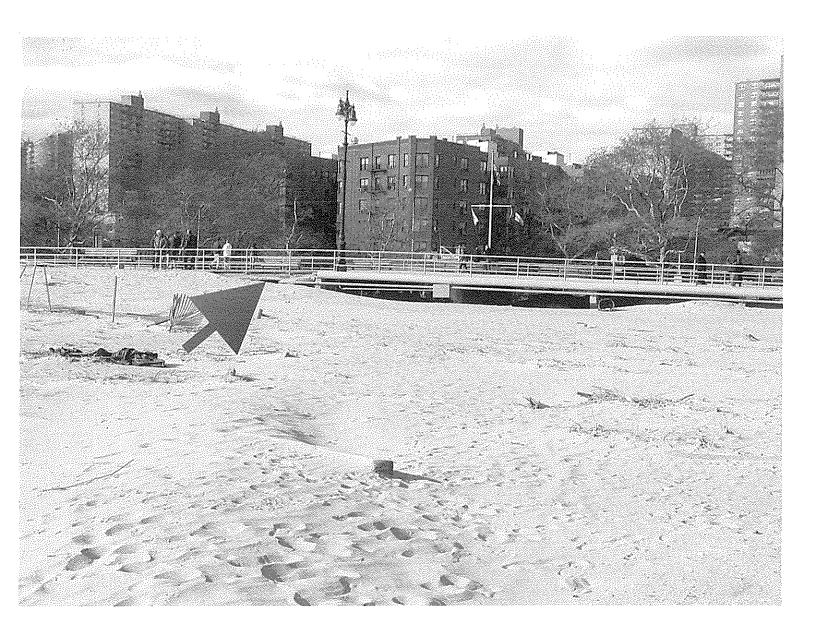
The line of demarcation is even more dramatic up close. The eroded area varied from 1-3 feet in height for the entire length of the concrete slab section, about three blocks.
